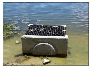
Stormwater Draiange Control Structure
